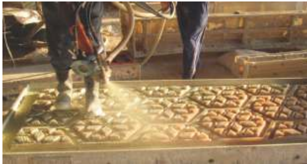
GFRC Casting with Spray Process
